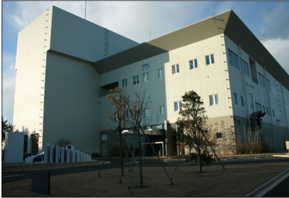
Materials and Life Science building, J-PARC.
